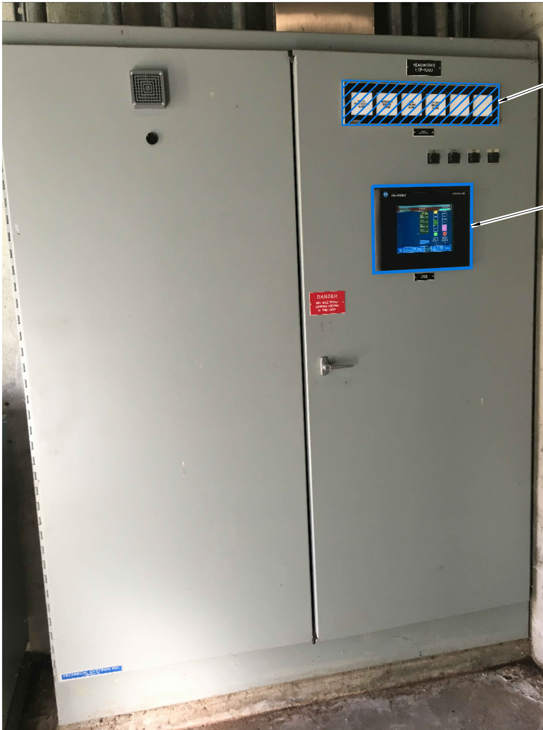
LCP-1000 EXTERIOR DEMO PHOTO
