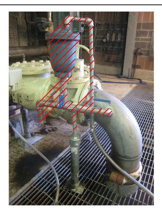
Remove air relief valve (at 3 REC pumps) and associated piping. Plug at 8" REC pipe. Pipe stand can be salvaged for roof vent pipe.
