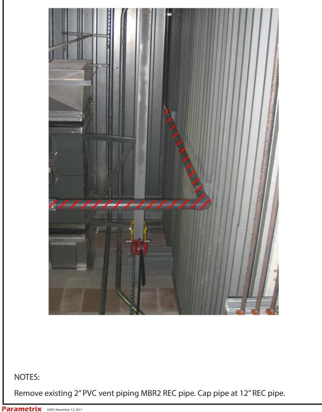
PHOTO 12 Removal of PVC Vent Pipe MBR2
