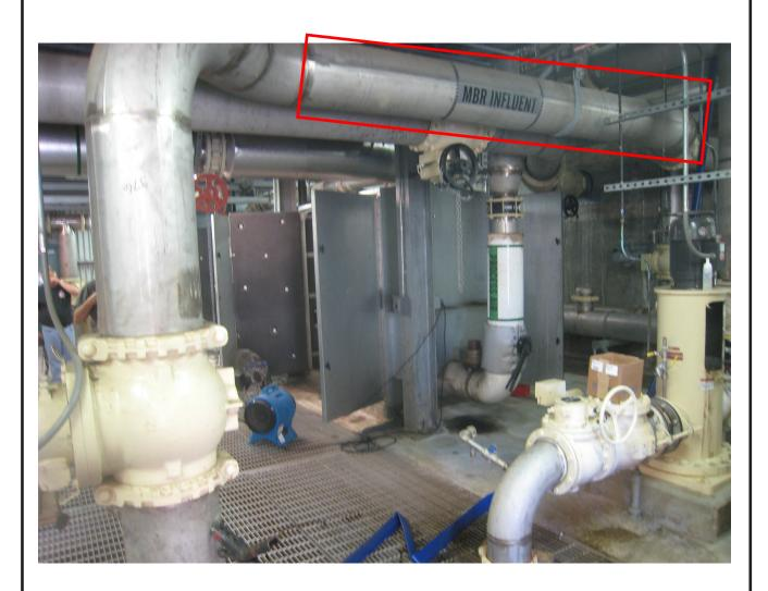
Lower existing 12" MBR1 pipes to MBR2 and MBR3 from  $\pounds$  elev 8.5 to  $\pounds$  elev 7.5. Existing 45° bends to be rotated per mechanical drawings.
