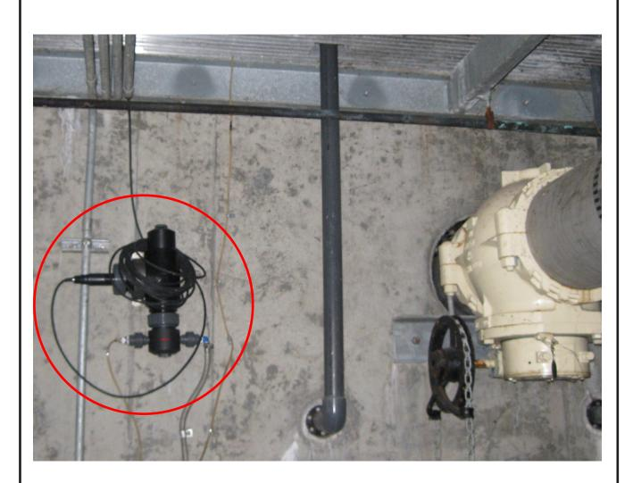
Move south turbidity meters from MBR2 and 3 to new location approximately 22' north to north end of the same 8" PERM pipe.
