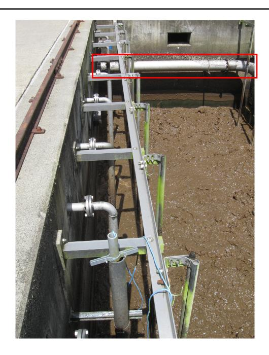
Move SST 10" PA to south end of MBR tank per mechanical drawings. Install cap on 10" PA where cut.
